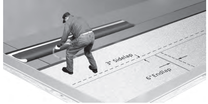
Figure 5-22: Remove the selvage edge release strip.
