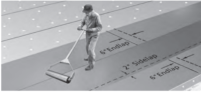
Figure 5-15: Roll seams with a heavy weighted roller.
